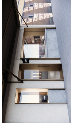
NEW SG-10 INTERNALLY ILLUMINATED BLADE SIGNAGE CONCEAL FIXED TO FACADE WALL. TEXT LUNE FINISH BLACK STEEL BACKINGS, WHITE ILLUMINATED TEXT
