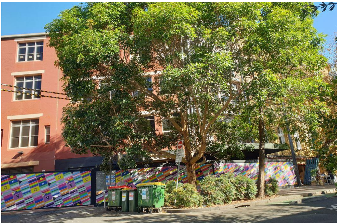
Figure 2: The northern Burton Street elevation (left) and north-eastern Foley Street elevation (right) of the lower ground floor level of the buildings at 56 and 58-60 Oxford Street, Darlinghurst respectively, viewed from the northern side of Burton Street, looking south
